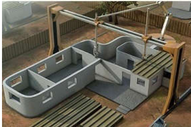
3D-Printer build a house
